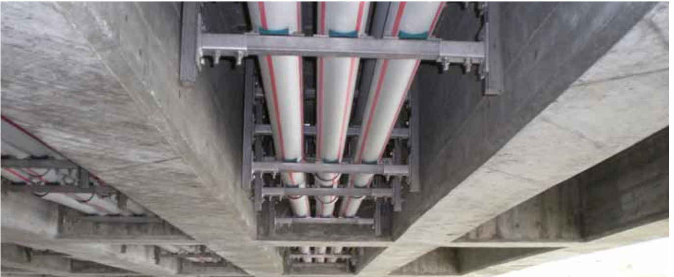
Drainage pipes installed with minimal drilling
