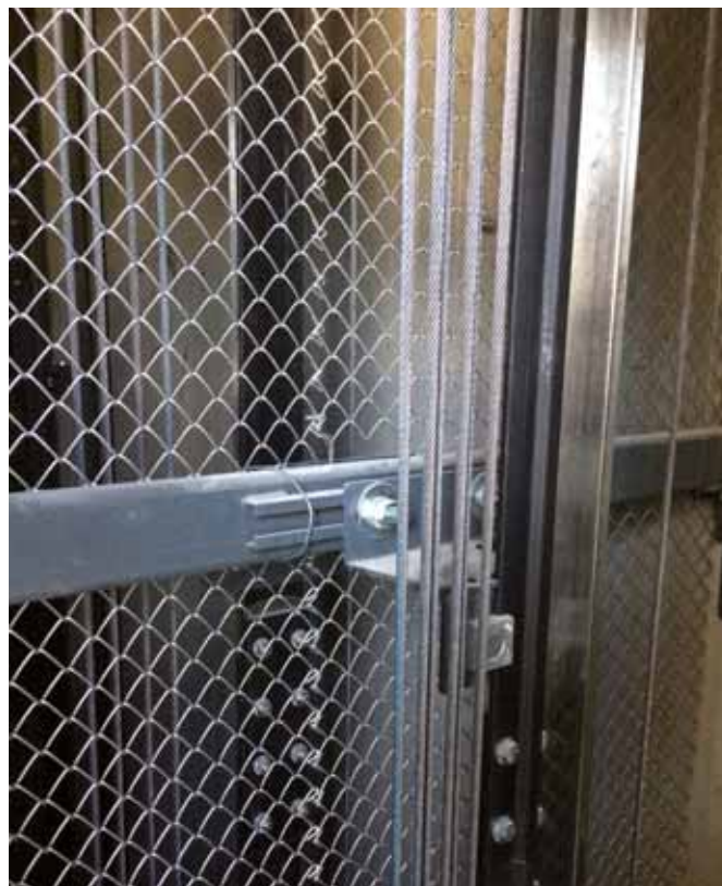
HALFEN Channels and bolts used in a lift shaft
