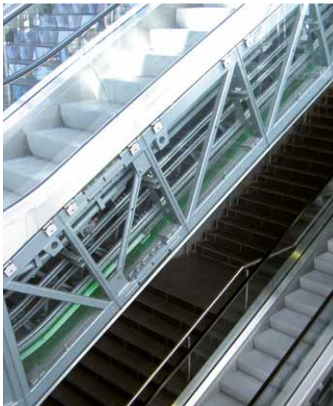
HALFEN Channels used in escalator construction
