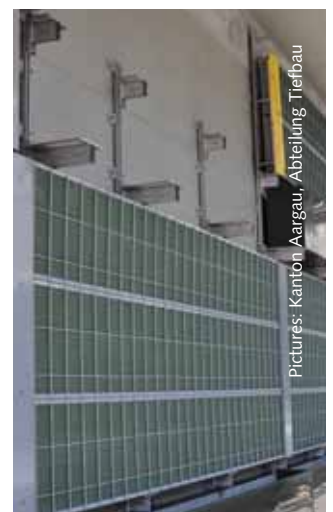
Noise reduction elements with planters mounted on easily adjustable brackets made of durable stainless steel
