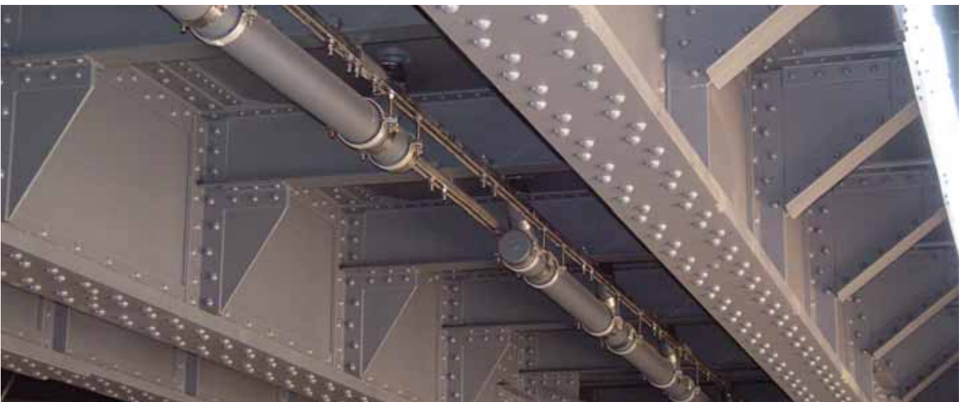
Upgrade and replacement of pipes without damaging bridge components and impacting the overall appearance
