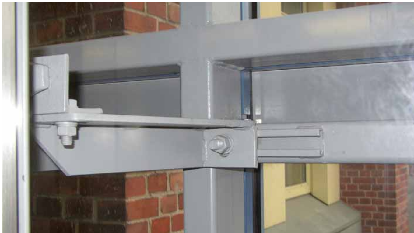
Adjustable connection on a steel frame
