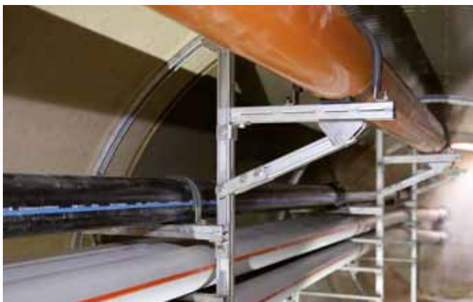
HALFEN Cantilevers as adjustable pipe supports
