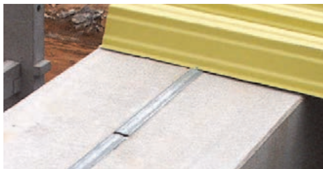
Fixing of trapezoidal sheet metal roof element
