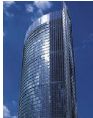
Post office Tower, Bonn
