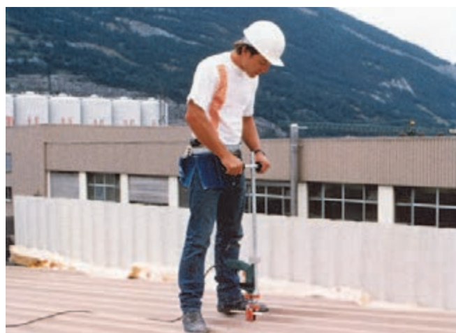
Fixing trapezoidal sheet metal using self-drilling screws
