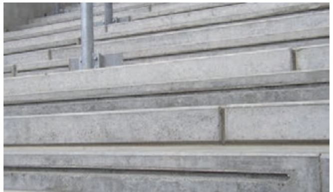
Fixing of safety rails, Rheinenergiestadion Cologne
