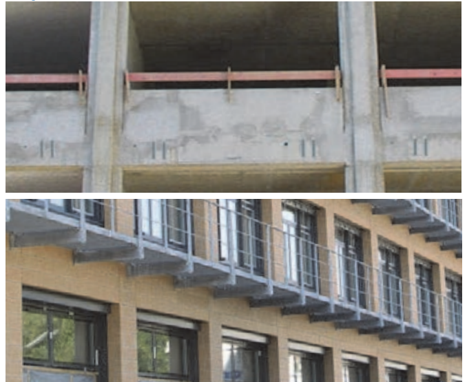
Fixings for emergency access balconies (Vertical installation of Halfen Channels)
