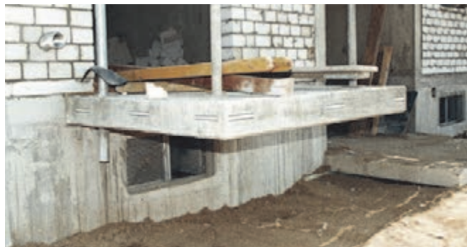
Cast-in HGB Channel, residential building
