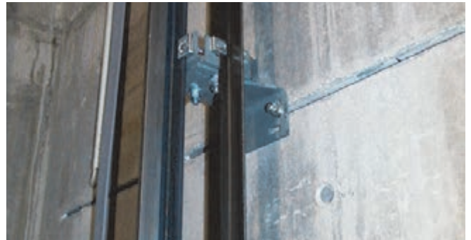
Fixing guide-rails with Halfen Channels
