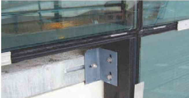
Fixings for curtain wall façades
