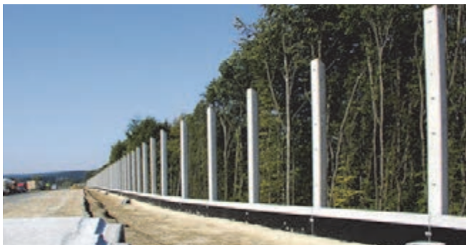
Fixings of noise barriers to concrete posts
