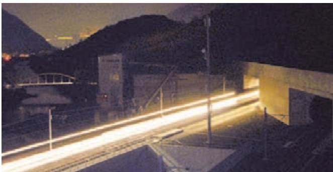
Lötschberg-Base tunnel, Switzerland
