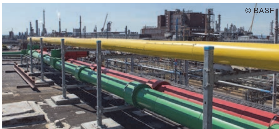
Typical application of the Halfen Powerclick system
