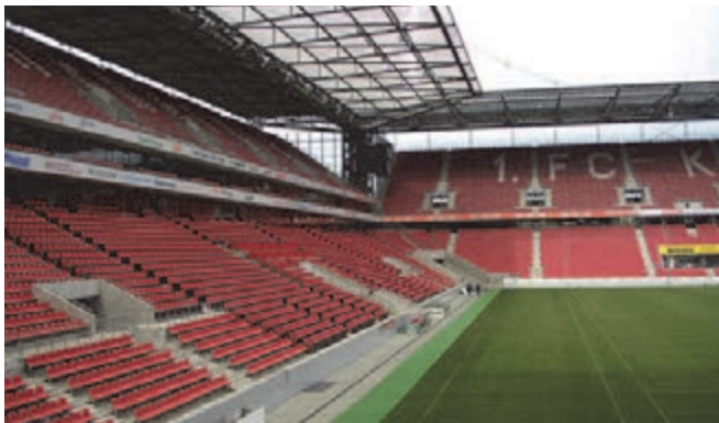
Fixing of safety rails, Rheinenergiestadion Cologne
