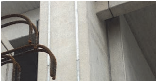
Vertical Halfen HTU Cast-in channels for fixing façade panels
