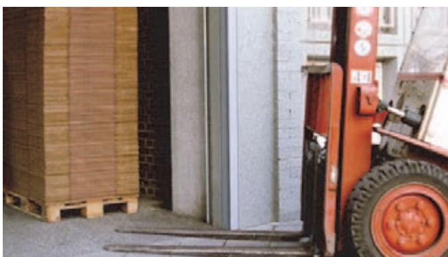
Corner guards in an industrial environment
