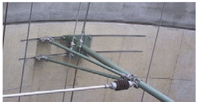
Fixing of overhead cables in railway tunnels
