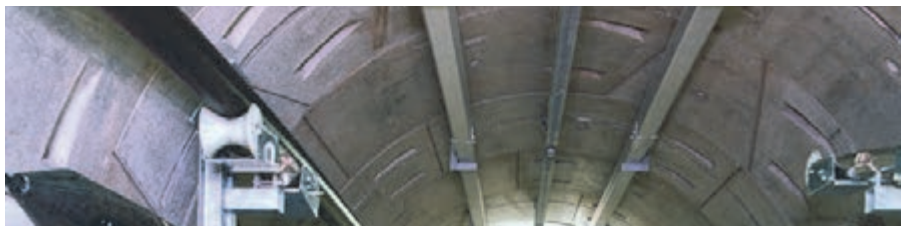
Curved Halfen Cast-in channels in tunnel segments
