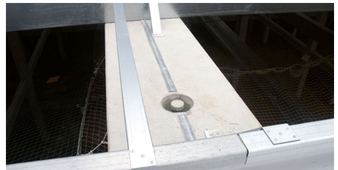
HALFEN HTU Cast-in channels in a pre-stressed concrete beam
