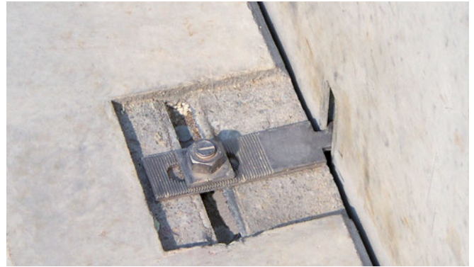
HALFEN HKZ Restraint tie with serrated washer
