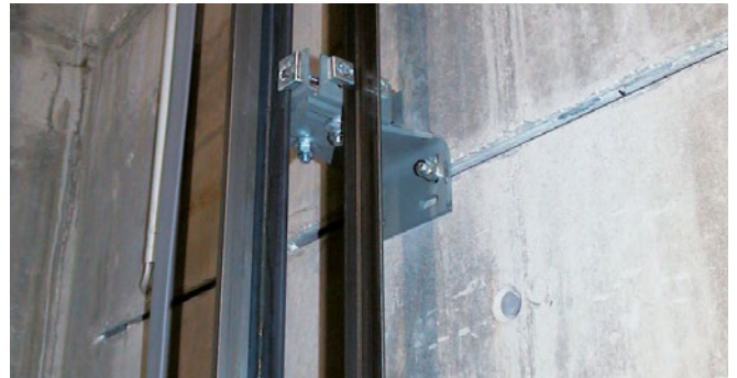
Fixing guide-rails with HALFEN Channels
