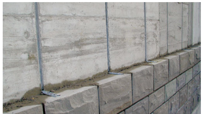
HALFEN ML Brick-tie anchor system
