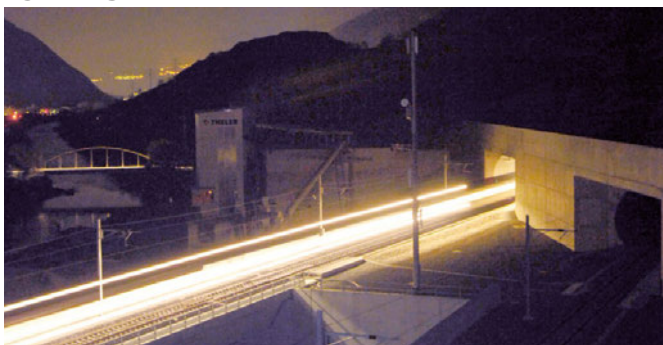
Lötschberg-Base tunnel, Switzerland
