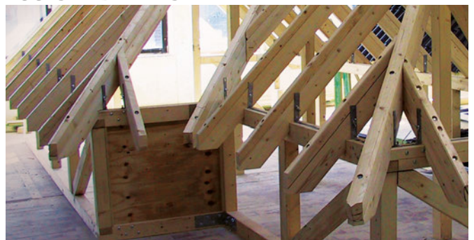
Timber pitched-roof construction
