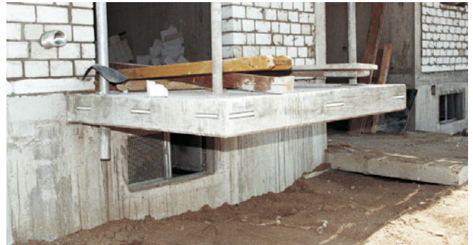
Cast-in HGB Channel, residential building
