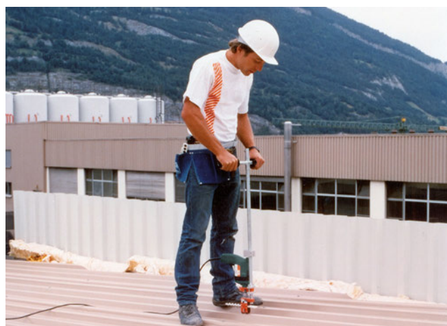
Fixing trapezoidal sheet metal using self-tapping screws
