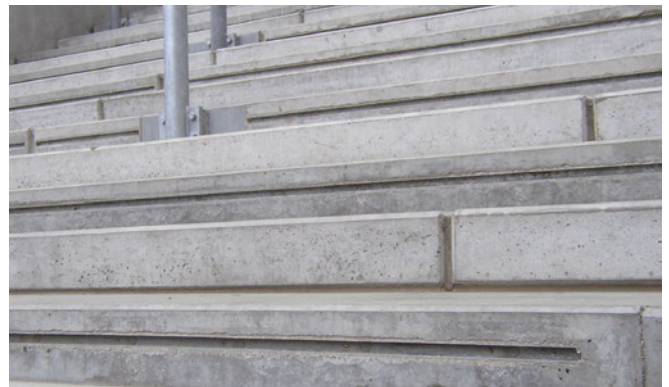
Fixing of safety rails, Rheinenergiestadion Cologne
