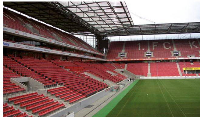
Fixing of safety rails, Rheinenergiestadion Cologne
