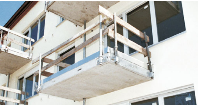
Used to secure safety rails during the construction phase
