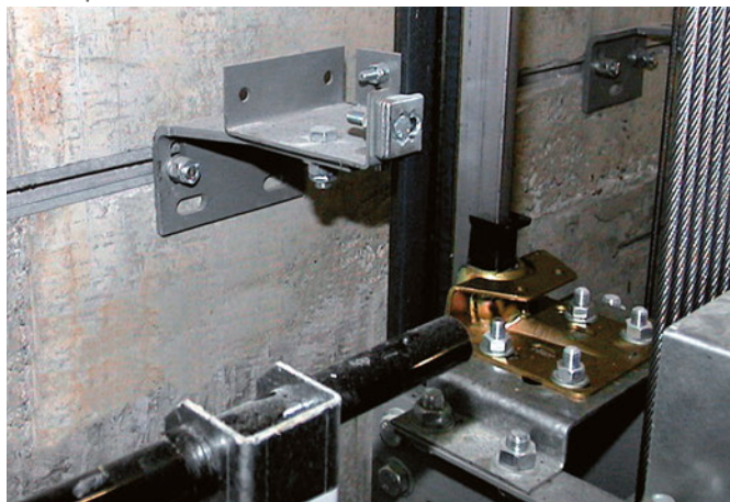
Fixing for guide-rails
