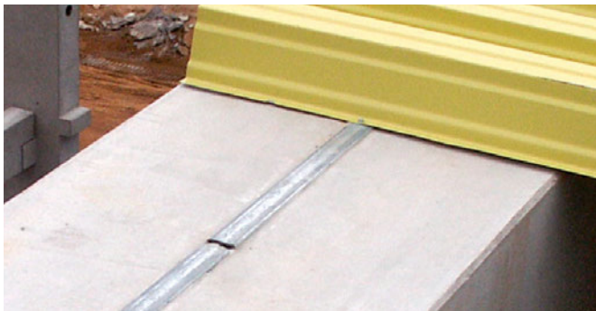
Fixing of trapezoidal metal sheeting roof element
