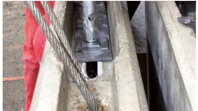
HVL-System in precast building components
