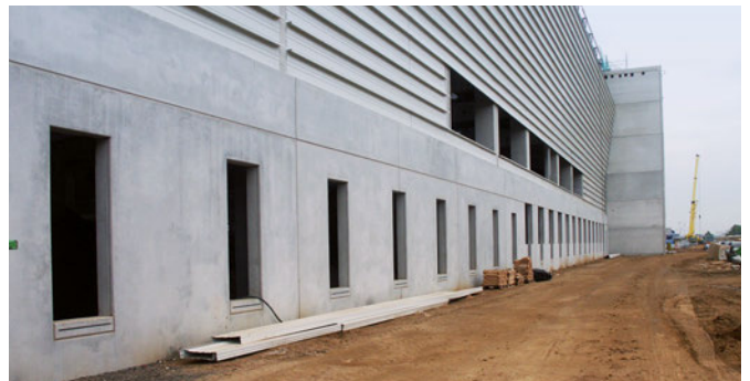
UPS Air Hub, Cologne Bonn Airport, Germany
