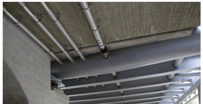
Fixings for drainage systems
