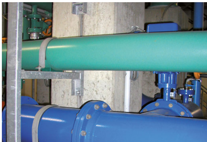
Pipe supports on vertical HZA Channels
