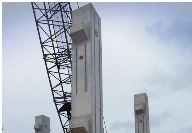
Vertical channels in columns to attach further components
