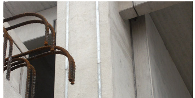
Vertical HALFEN HTU Cast-in channels for fixing façade panels
