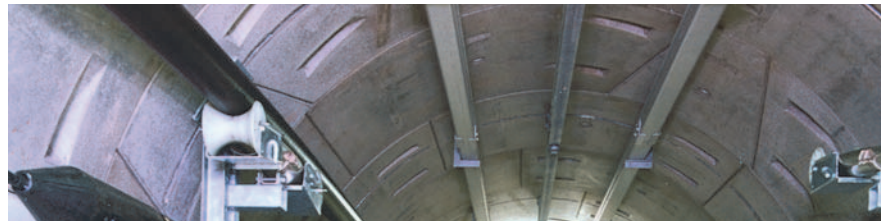
Curved Halfen Cast-in Channels in tunnel segments
