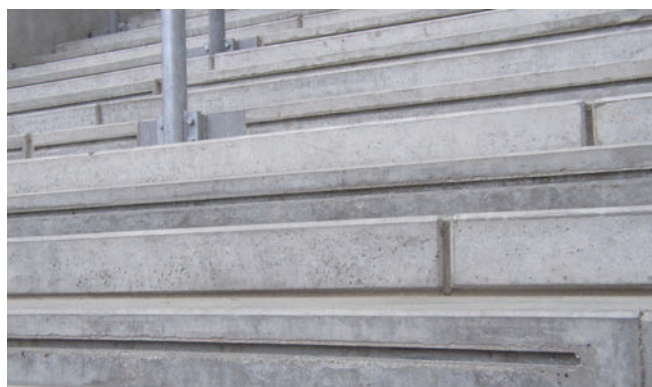
Fixing of safety rails, Rheinenergiestadion Cologne
