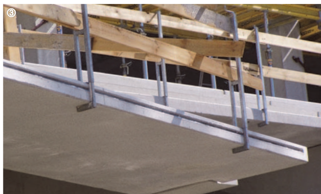
①-④: Safety barrier installation, multi purpose arena in Berlin
