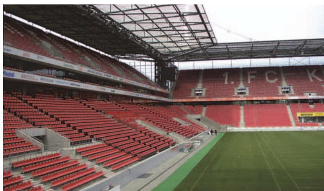
Fixing of safety rails, Rheinenergiestadion Cologne
