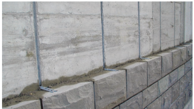
Halfen ML Brick-tie anchor system
