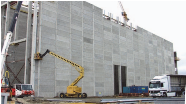
HVL-System application; precast components installed between the columns; Airbus paintshop building
