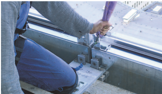
Fixing of a modular façade using HCW-ED Brackets on HTA-CE Anchor Channels
