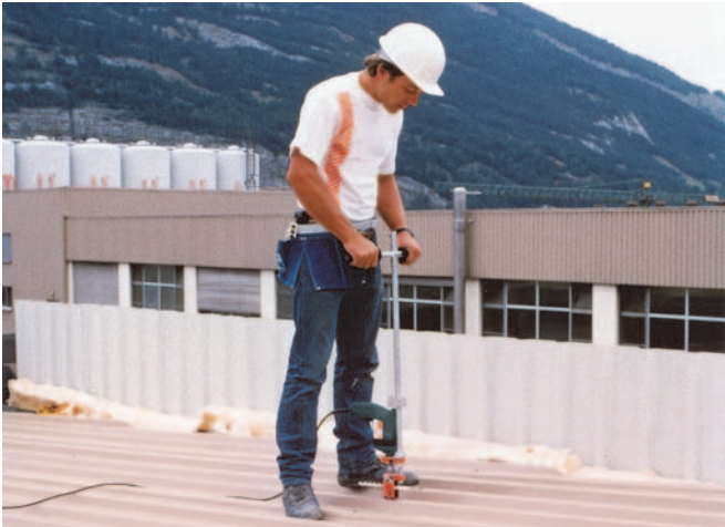
Fixing trapezoidal sheet metal using self-drilling screws
