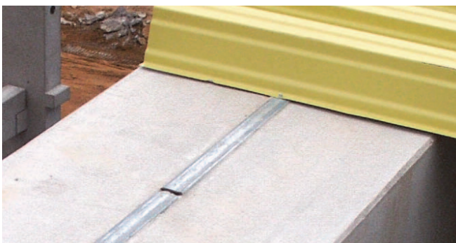
Fixing of trapezoidal sheet metal roof element
